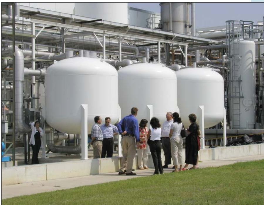
**Water Conservation Division's Bill Hoffman escorts a tour group through Samsung's on-site water reuse facilities. The recycled water system supplies all of Samsung's landscape water, up to 125,000 gpd, and reduces wastewater discharge by more than 250,000 mgd. The plant currently recycles more than 60% of the water it uses.**
