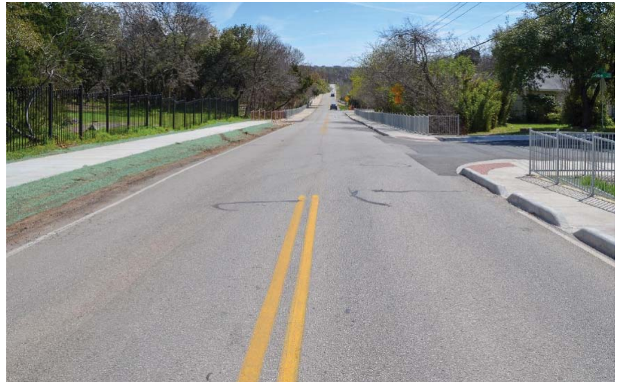
GABLE DRIVE AFTER
