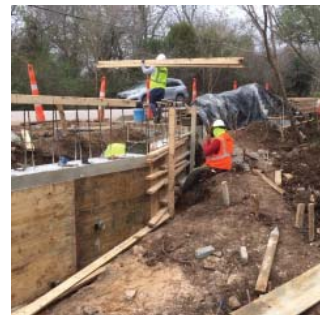
ADELPHI LANE CREEK CROSSING DRAINAGE CONSTRUCTION
