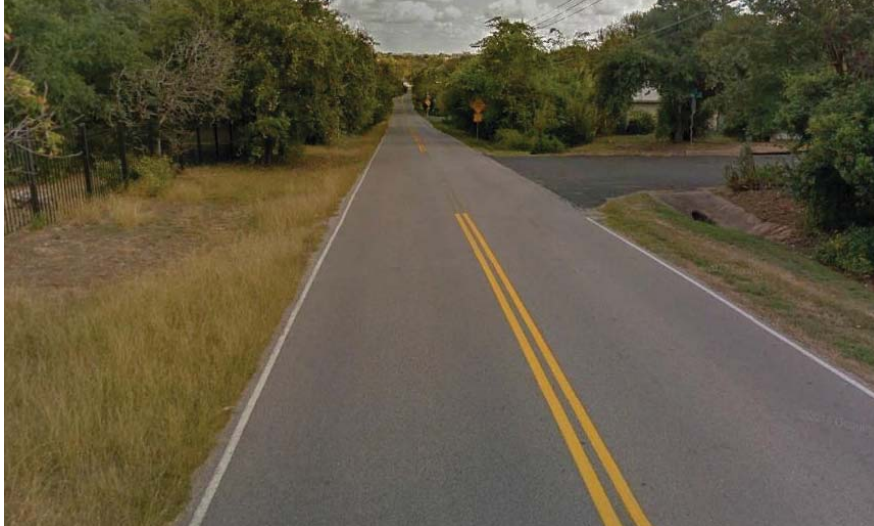
GABLE DRIVE BEFORE
