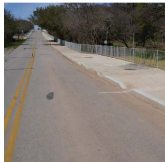
ADELPHI LANE CREEK CROSSING AFTER
