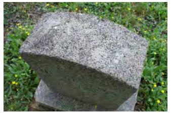
Figure 317. Concrete grave marker with distinctive mica aggregate (McDoux Preservation)
