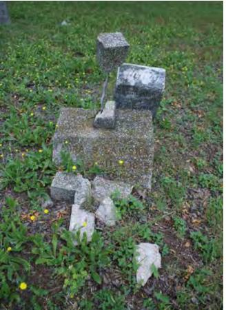
Figure 322. Broken concrete cross (McDoux Preservation)
