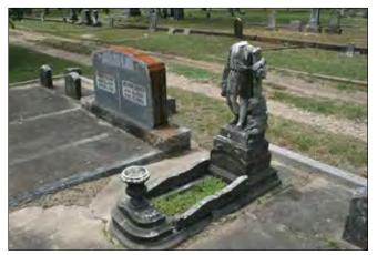
Figure 103. Cradle marker; the head of the statue has been broken off. (John Milner Associates)
