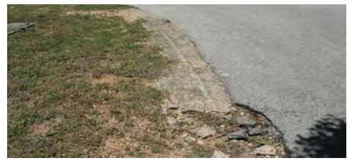
Figure 355. Edge degradation of the cemetery drive due to vehicle parking (John Milner Associates)
