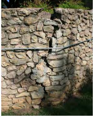
Figure 536. Severely cracked portion of the wall, with attempted repair visible below the steel conduit (John Milner Associates)
