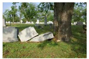
Figure 261. Marker displaced by adjacent tree roots (McDoux Preservation)
