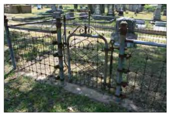
Figure 173. Woven wire fencing surrounding a family plot (John Milner Associates)
