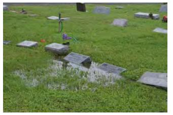
Figure 511. Ponding and subsidence in Section 7 (McDoux Preservation)
