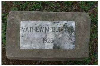
Figure 318. Stone marker enframed in concrete (McDoux Preservation)
