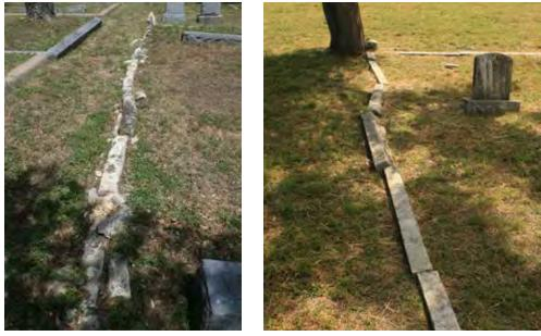
Figure 162. (left) Severely damaged limestone curb, probably due to mowers; (right) displaced curbing (John Milner Associates)
