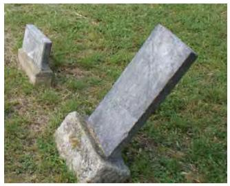
Figure 267. Severely tilted marker (McDoux Preservation)
