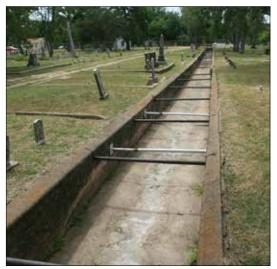
Figure 179. The concrete drainage channel that bisects the cemetery (John Milner Associates)
