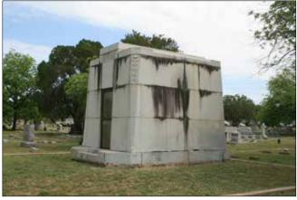
Figure 192. Hamilton mausoleum in Section 3, with some staining and an exposed foundation (John Milner Associates)
