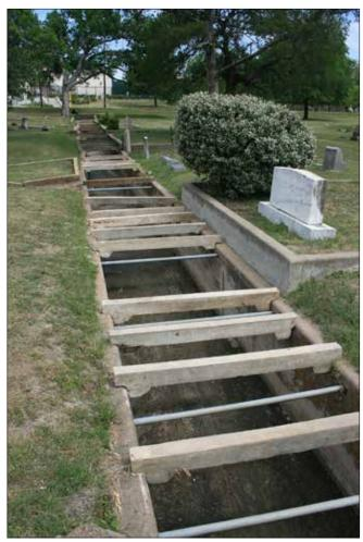
Figure 183. Cast concrete and iron pipe spacers stabilize the channel in the northern portion of the cemetery. (John Milner Associates)
