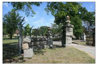
Figure 200. Several blocks on the north wing wall of the west entrance are displaced. (John Milner Associates)
