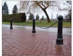
Figure 221. Steel bollards with chain (RelianceFoundry.com)
