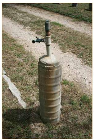
Figure 187. Iron pipe riser with hose bib (John Milner Associates)
