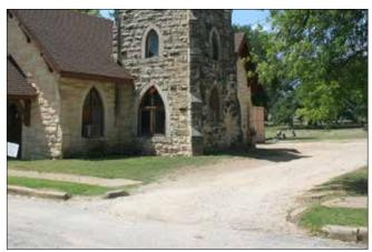
Figure 66. The curb at the intersection adjacent to the chapel is extremely degraded. (John Milner Associates)
