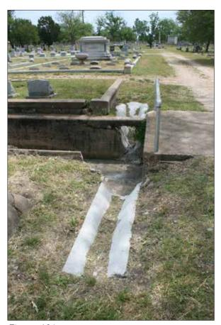
Figure 186. Concrete swales added to mitigate erosion (John Milner Associates)
