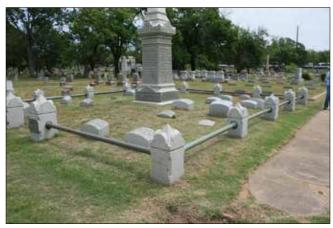
Figure 175. Gas pipe fencing set in stone piers (John Milner Associates)
