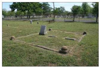
Figure 154. Poured concrete curb with decorative corner piers (John Milner Associates)
