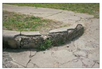
Figure 65. Turning vehicles have caused severe damage to this curb. (John Milner Associates)
