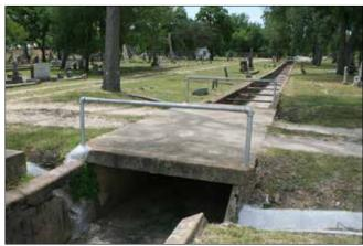
Figure 61. A concrete vehicular bridge crossing the drainage channel (John Milner Associates)
