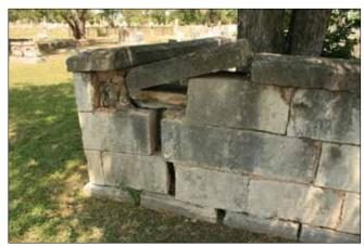
Figure 165. The wall is severely cracked, and has missing and displaced stones. (John Milner Associates)
