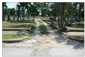
Figure 72. The north-south gravel roads are often in especially poor condition near their intersections with Main Avenue. (John Milner Associates)
