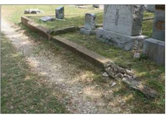
Figure 73. Eroded road beds are causing adjacent features to lean and break, as is visible in the curbing here. (John Milner Associates)
