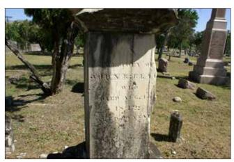
Figure 128. Damaged limestone tablet (McDoux Preservation, OW-DSC00051)
