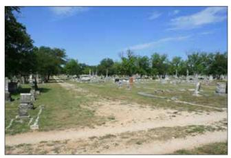
Figure 71. This drive has lost much of its gravel surfacing. (John Milner Associates)
