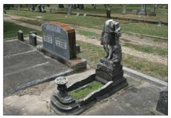
Figure 103. Cradle marker; the head of the statue has been broken off. (John Milner Associates)
