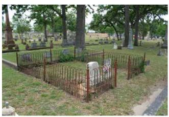
Figure 169. Bent metal fencing (John Milner Associates)
