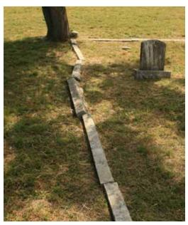
Figure 162. (left) Severely damaged limestone curb, probably due to mowers; (right) displaced curbing (John Milner Associates)
