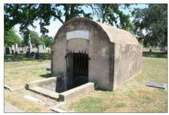
Figure 195. The concrete-stucco-clad, brick masonry Kreisle mausoleum in Section 1 (John Milner Associates)
