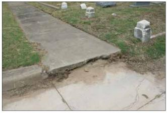
Figure 68. Severe displacement where the sidewalk crosses a cemetery road (John Milner Associates)
