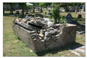
Figure 143. Deteriorated brick tomb (John Milner Associates)
