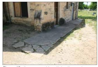
Figure 69. A concrete sidewalk leading to the chapel restroom is similarly in poor condition. (John Milner Associates)
