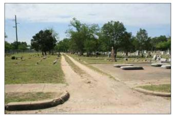
Figure 70. Gravel washes off the road surface, collecting at the road margin. (John Milner Associates)
