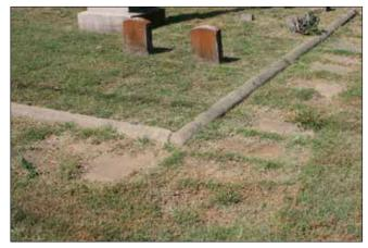
Figure 74. Grass intruding on a paved path has obscured the paving stones. (John Milner Associates)
