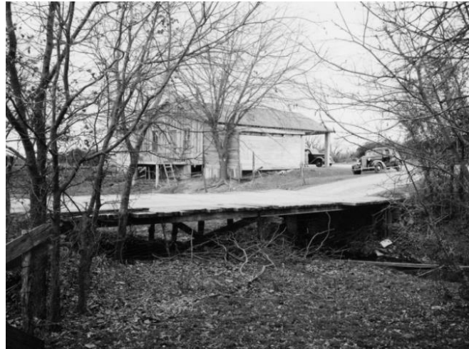
North Loop at Burnet Road (City of Austin,
