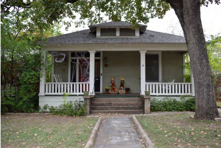
Fig. 4-2-2. Example of a 1914 National Folk house with a square-plan hipped-roof square-plan form located at 300 W. 35th Street. Note the horizontal siding, door with transoms, and lack of applied ornament. Source: Photo by HHM, 2019.
