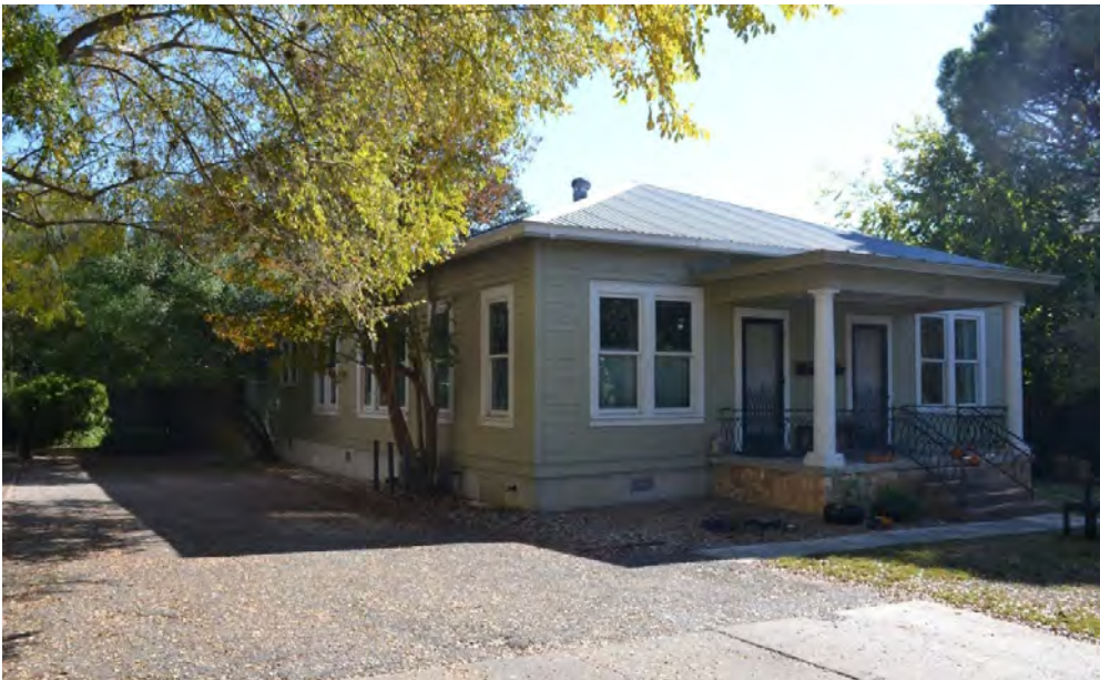
Figure 5-4-6. Oblique view of the home at 1909 Cliff Street (1925), which was originally a single-family home but was later converted into a duplex. Source: HHM, 2019.
