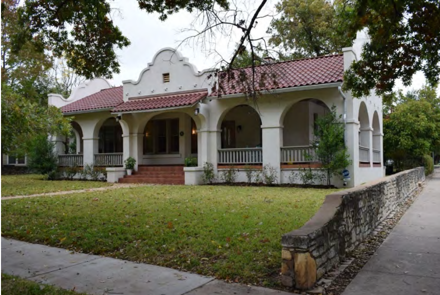
Figure 5-2-12. Oblique view of the home at 3001 Washington Square (1912), one of the stately and suburban-style homes in the Washington Square development. It is an example of the Mission Revival style sparsely present in the district. Source: HHM, 2019.
