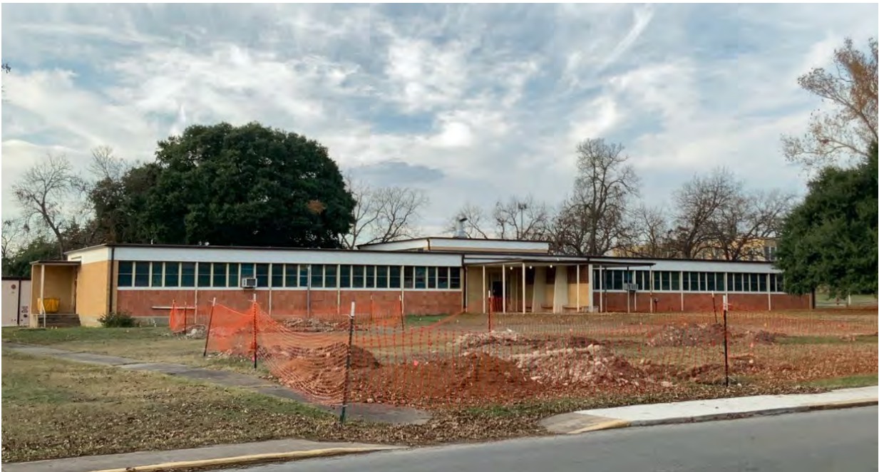
Figure 5-3-9. Oblique view of the 1952 African American Dining Hall (Building 736), demolished in 2020. This was one of the few buildings on the hospital campus constructed specifically to serve the segregated patient population. Source: HHM, 2019.
