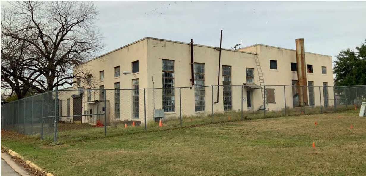
Figure 5-3-6. Oblique view of the 1899 steam-powered electrical plant (Building 538), which allowed the facility greater self-sufficiency and independence from the City of Austin. Source: HHM, 2019.
