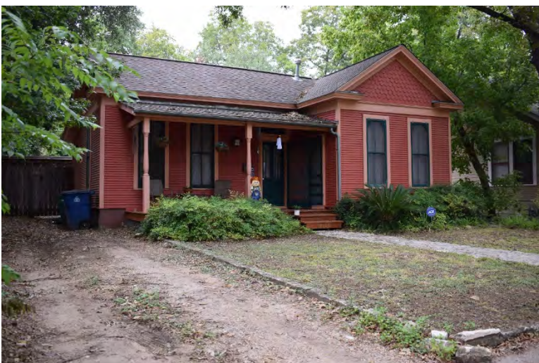
Fig. 4-2-4. Example of a 1910 Folk Victorian house with a L-plan form located at 4506 Avenue G. Source: Photo by HHM, 2019.
