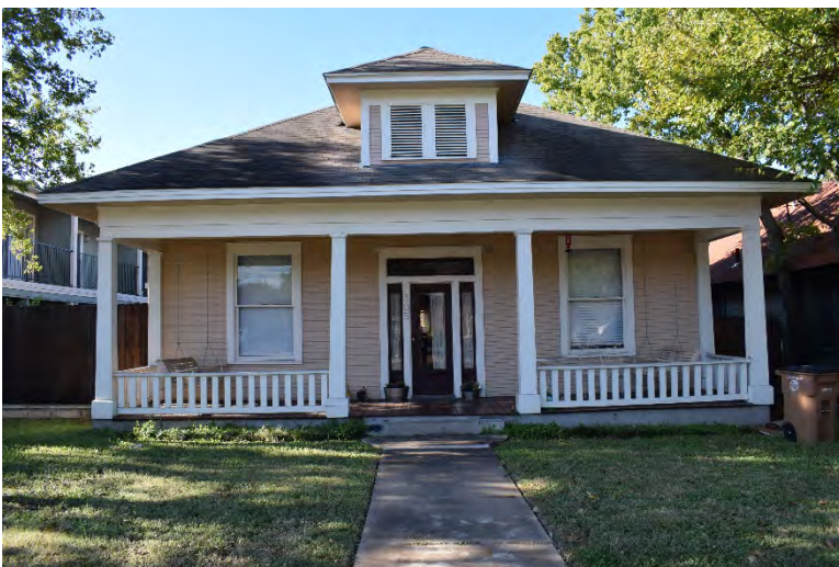
Fig. 4-1-6. The square-plan hipped-roof form is a common domestic house type in North Central Austin, and this example at 305 W. 38th Street exhibits many common physical features of the form. Constructed in 1917, this dwelling has a low-pitched hipped roof with a centrally located, low-pitched hipped-roof dormer on the front.
