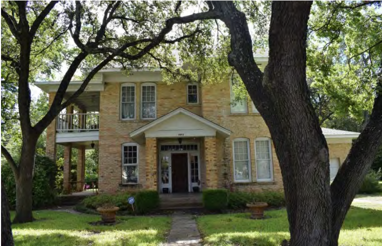
Figure 5-10-6. Façade of the Tadlock-Brownlee-Harris House (1913) at 1901 West 35th Street. Source: HHM, 2019.
