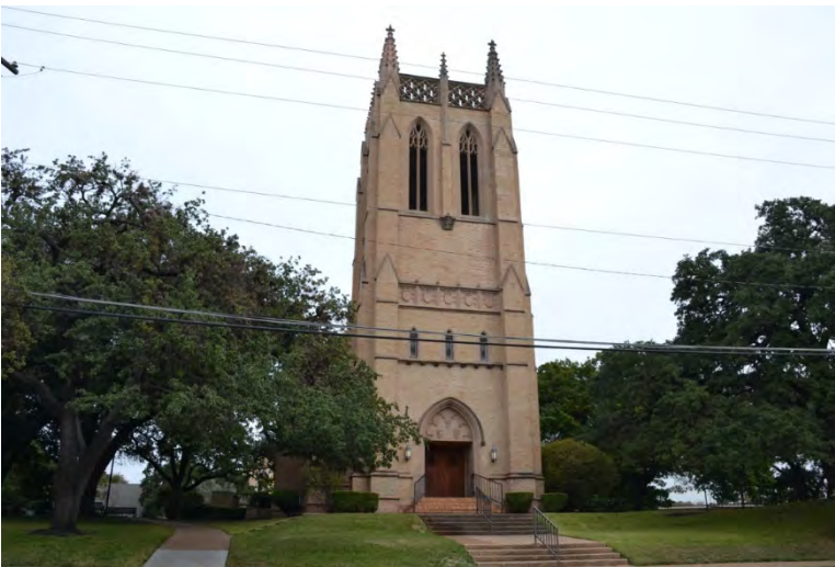
Figure 5-12-6. Façade view, facing north, of the ca. 1941 Gothic Revival Shelton Chapel on the Austin Presbyterian Seminary Campus. Source: HMM , 2019.
