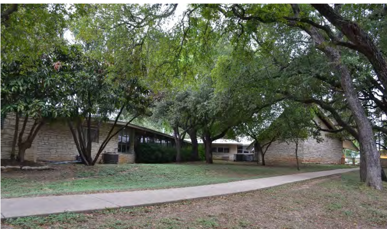
Fig. 4-1-42. These buildings populate the St. Andrews Episcopal School campus, located at 3104 Wabash Avenue. They serve as examples of private school buildings in the North Central Austin Survey Area. The 1957 buildings exhibit Mid-century Modern style influences. Source: Photo by HHM, 2019.
