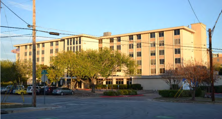
Fig. 4-1-38. This hospital building, which houses Seton Hospital, is located at 3501 Mills Avenue and was constructed in 1959. The six-story edifice features a vertical-block building form with minimal architectural stylistic influences. Note the ample parking spaces surrounding the hospital building. Source: Photo by HHM, 2019.
