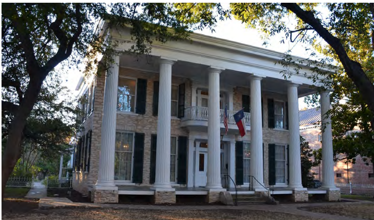
Figure 5-1-2. Neill-Cochran House (1855) at 2310 San Gabriel Street. Source: HHM, 2019.
