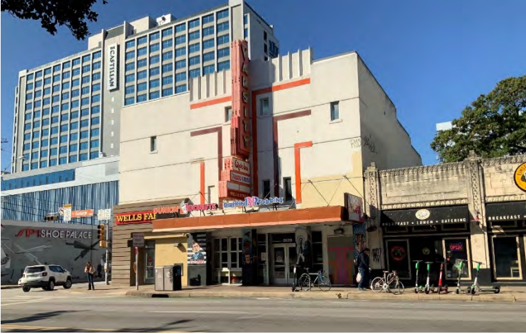
Fig. 4-2-8. Photo of the 1936 movie theater at 2402 Guadalupe Street exhibiting bold and colorful Art Deco detailing. Note the decorative motif in the parapet and projecting marquee. Source: Photo by HHM, 2019.
