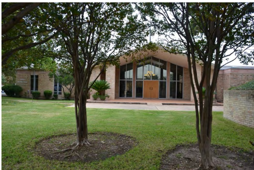
Figure 5-12-9. Façade view of the 1961 Trull Administration Building, including its Mid-century Modern entranceway. Source: HHM, 2019.
