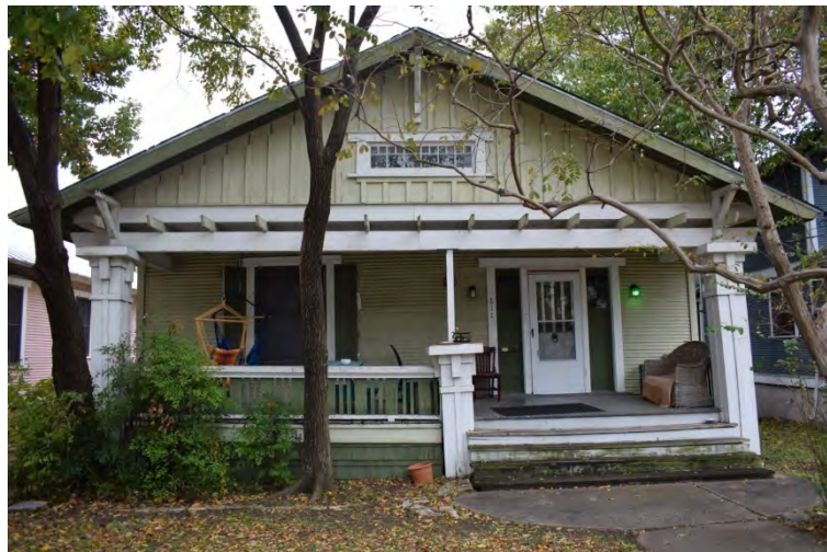
Figure 5-2-11. Façade view of the Craftsman bungalow home at 611 West 31st 1/2 Street (1920). This is an example of a common form and style developed throughout the district during the 1920s and 1930s. Its neighbors share the same footprint and stylistic influences, all of which were built in the first years of the 1920s, per Sanborn maps. Source: HHM, 2019.
