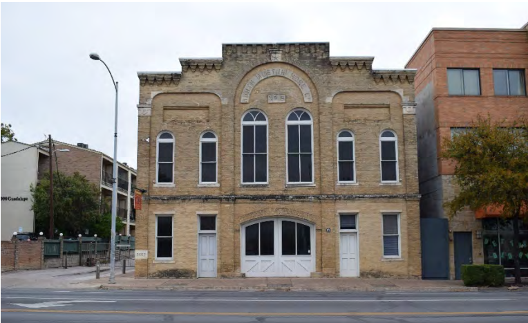
Fig. 4-1-44. This is an example of a fire station in the North Central Austin survey area. It is located at 3002 Guadalupe Street and has a two-part commercial block form with Italianate stylistic detailing. Note the three enclosed bays across the front façade. Source: Photo by HHM, 2019.
