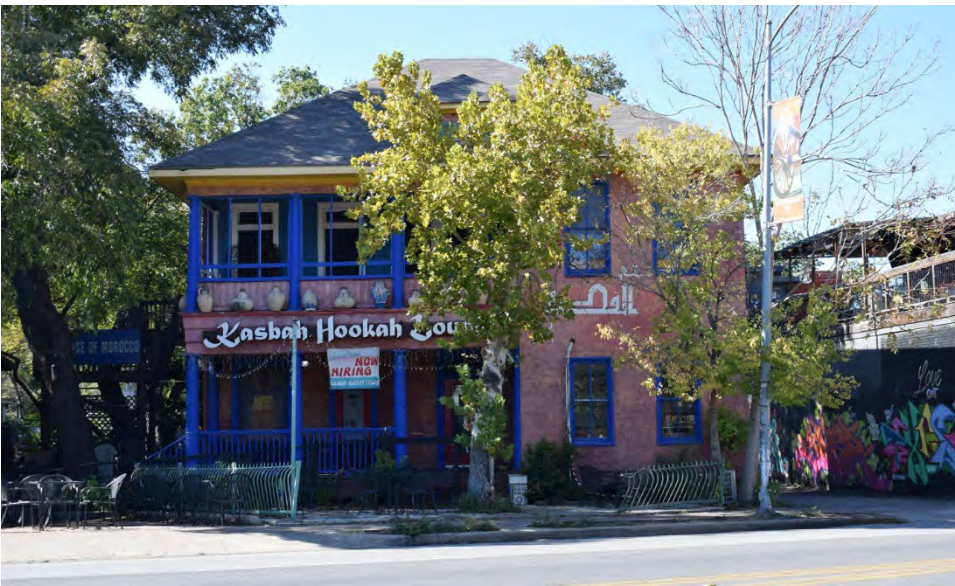
Figure 5-7-2. Façade of the house at 2714 Guadalupe Street (1900). Source: HHM, 2019.
