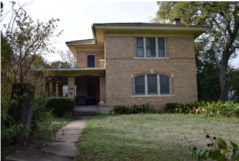
Fig. 4-2-10. Photo of a 1922 Prairie style house, located at 609 W. 32nd Street. Note the brick exterior, use of a belt course, and low-sloping eaves. Source: Photo by HHM, 2019.
