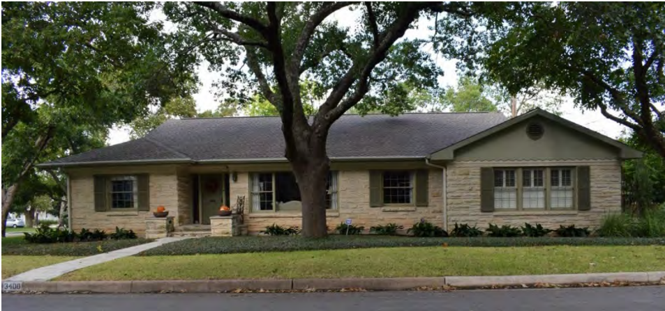
Figure 5-10-11. Façade of the Minimal Traditional ranch house (1949) at 3400 Happy Hollow. Source: HHM, 2019.
