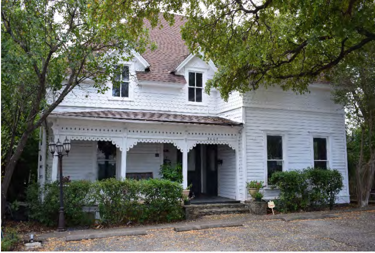
Fig. 4-1-5. This example of a Folk -Victorian style house with a modified L-plan form is located at 3406 Glenview Avenue and was constructed about 1910. Its steeply pitched roof and extending cross gables are hallmarks of the modified L-plan form. Source: Photo by HHM, 2019.
