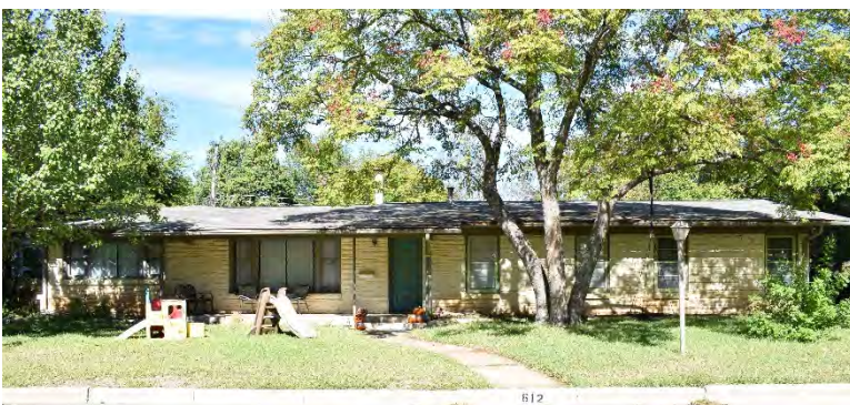
Fig. 4-1-12. Example of a house with a ranch form located at 612 E. 48th Street. This one-story house has many features typical of the Ranch style, including a low-slung profile, large picture window, wide overhanging eaves, and brick-veneered exterior. Source: Photo by HHM, 2019.
