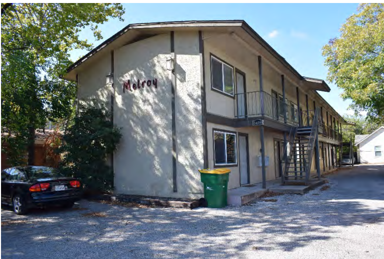
Fig. 4-1-22. This example of a linear low-rise apartment building is located at 3408 Speedway and was constructed in 1972. The long, rectangular, two-story building has a linear configuration with balconies and exterior staircases running along the side. Source: Photo by HHM, 2019.
