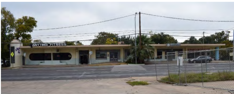
Fig. 4-2-9. Building with Streamline Moderne stylistic influences at 3401 Guadalupe Street. Note the horizontal emphasis, cantilevered awning, and oval-shaped windows. Source: Photo by HHM, 2019.
