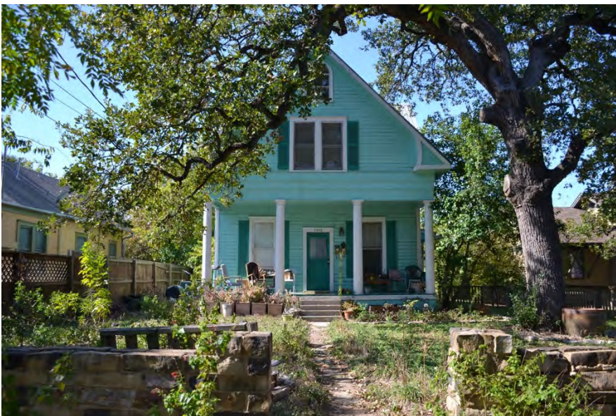
Figure 5-6-7. Façade of Colonial Revival house (1910) at 3408 Cedar Street. Source: HHM, 2019.
