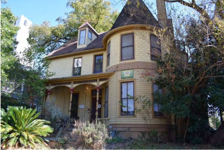
Fig. 4-2-5. Oblique view of 1882 a Queen Anne house at 1909 Nueces Street. Note the spindle work and turned- wood columns on the porch, hipped-roof dormer, and cupola-topped turret. Source: Photo by HHM, 2019.
