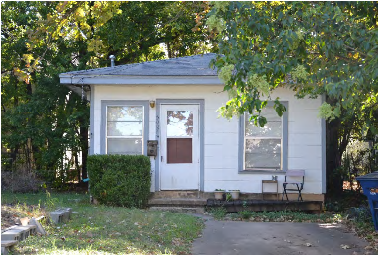
Fig. 4-1-16. This example of a back house is located at 5007 Rowena Street. Constructed in 1948, this back house is situated at the rear of the main house. It is a one-story rectangular building with a hipped roof. Source: Photo by HHM, 2019.
