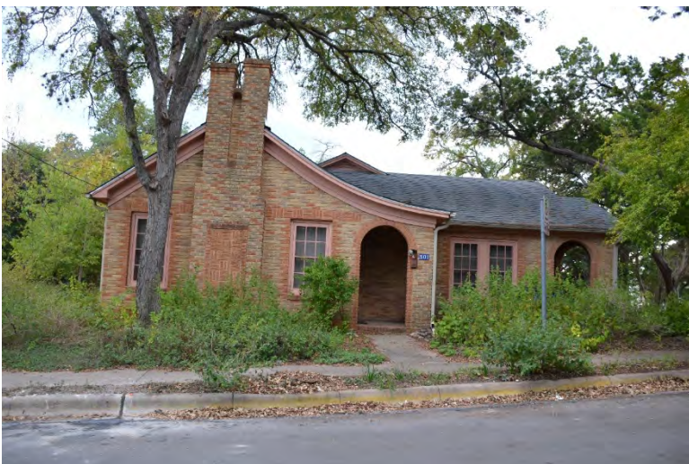
Fig. 4-2-12. Example of a brick Tudor Revival house at 301 Moore Boulevard. Note the use of the bungalow form with Tudor Revival stylistic details like its round-arched door and broad chimney. Source: Photo by HHM, 2019.
