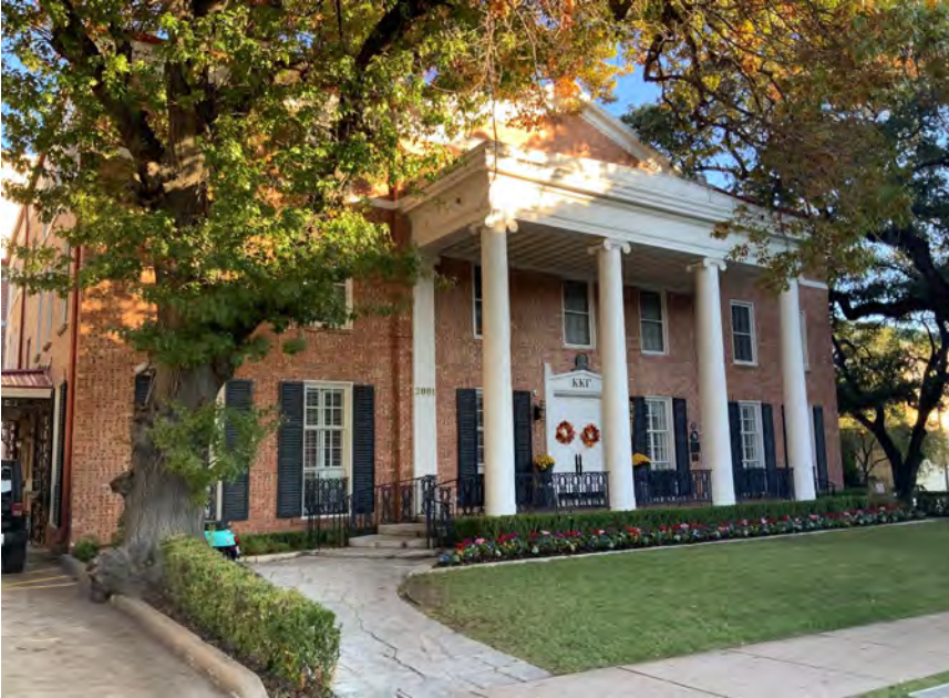
Figure 5-1-24. Kappa Kappa Gamma Sorority House at 2001 University Avenue (built around 1930). Source: HHM, 2019.
