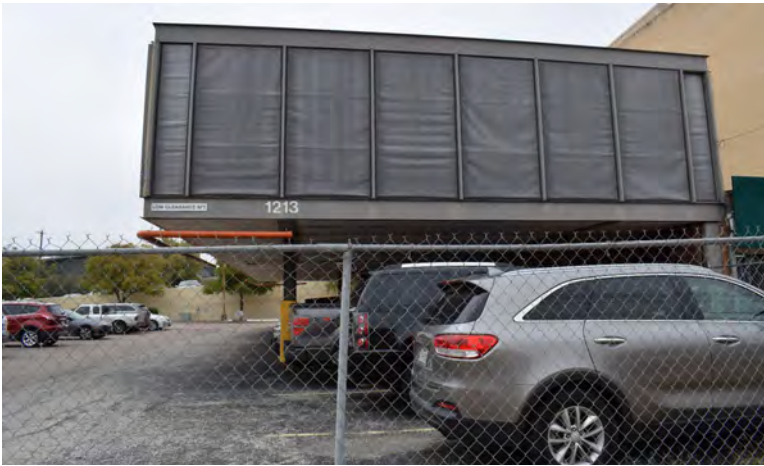
Fig. 4-1-32. This is an example of a raised box property at 1213 W. 34th Street. Note the open space used as a parking garage beneath the raised building. This building takes up a small footprint of the lot in order to allow for parking on the side of, under, and in front of the building. The Modern style reflects the mid-century period in which the building was constructed. Source: Photo by HHM, 2019.
