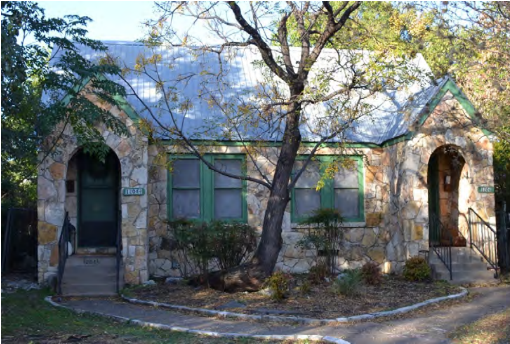
Fig.5-4-5. Photo of the ca. 1935 duplex at 1204 West 22nd Street. Source: Photo by HHM, 2019.
