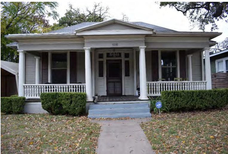
Fig. 4-1-2. Example of a center-passage house located at 608 W. 31 ½ Street. This house, constructed in 1915, has many typical features of a one-story center-passage house, including a centralized entryway and a mostly symmetrical façade. Like many examples within the North Central Austin survey area, this house has an inset porch along the front façade. The Classical columns and turned-wood balustrade that articulate the porch and the pronounced cornice are indicative of Classical Revival traditions, a popular architectural expression in Austin during the early twentieth century. Source: Photo by HHM, 2019.
