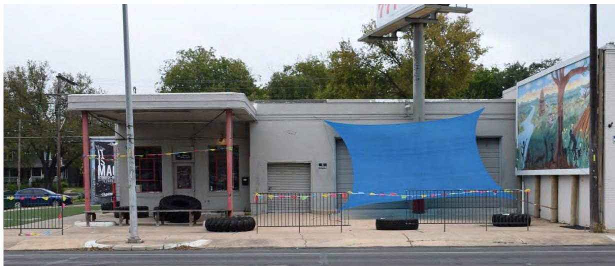
Figure 5-5-8. Façade of the former gas station at 4227 Guadalupe Street (1942). Source: HHM, 2019.
