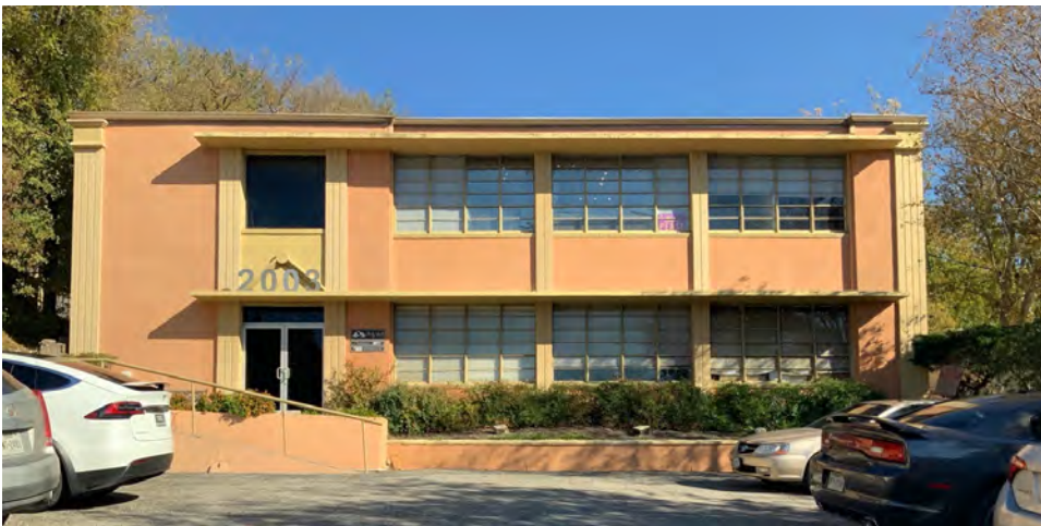
Figure 5-4-11. Façade view of the 1962 two-story office building constructed at 2003 North Lamar Boulevard. Designed with ample parking in front, this property is an example of commercial building types found along major roadways within the district around the mid-twentieth century. Source: HHM, 2019.
