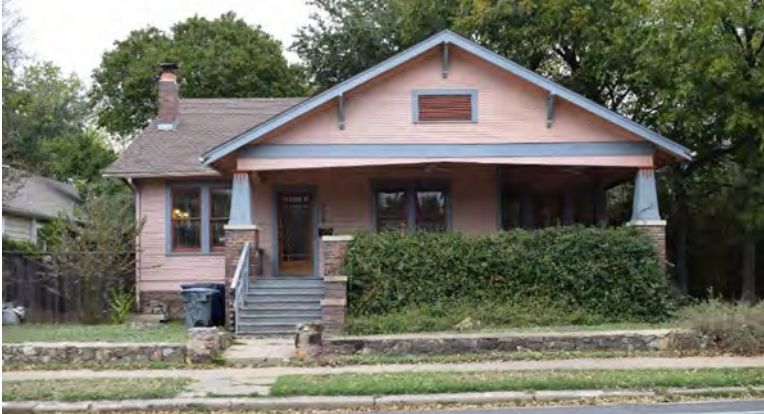
Fig. 4-2-11. Photo of a 1922 Craftsman house, located at 904 W. 29th Street. Note the horizontal emphasis with broad eaves and paired windows. Also note the brick pedestals, tapered columns, and wood brackets. Source: Photo by HHM, 2019.
