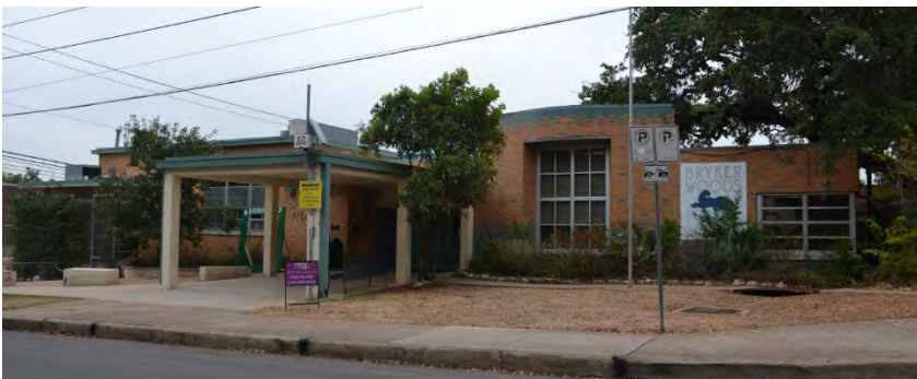
Figure 5-10-7. View of Bryker Woods Elementary School (1939) at 3309 Kerbey Lane. Source: HHM, 2019.
