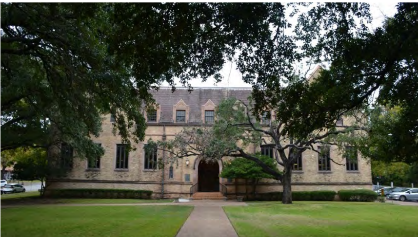
Figure 5-12-7. Façade view of Stitt Library, which was constructed in 1945 adjacent to Shelton Chapel. Source: HHM, 2019.
