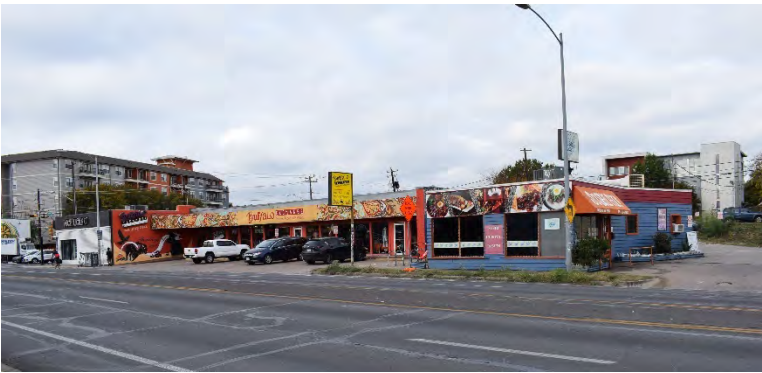
Fig. 4-1-34. Example of a commercial strip at 2904 Guadalupe Street, constructed in 1949. Source: Photo by HHM, 2019.
