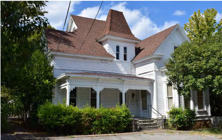
Figure 5-1-21. Photo of the Champion house at 3406 Glenview Avenue, which originally was on a large parcel of land closer to Shoal Creek. The house was relocated here around 1939 to facilitate realignment of West 34th Street and construction of a bridge over Shoal Creek. Source: HHM, 2019.
