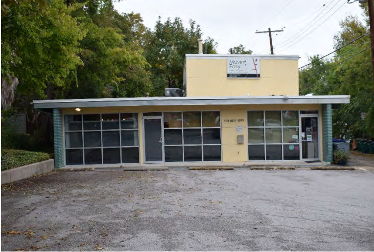
Fig. 4-1-30. This is an example of a commercial box property at 404 W. 30th Street. Note the wide, overhanging eaves on the front and side that would cover a person as they left their car and walked into the building. This building takes up a small footprint of the lot in order to allow for parking on the side of and in front of the building. The distinct Mid-century Modern style reflects the mid-century period in which the building was constructed. Source: Photo by HHM, 2019.
