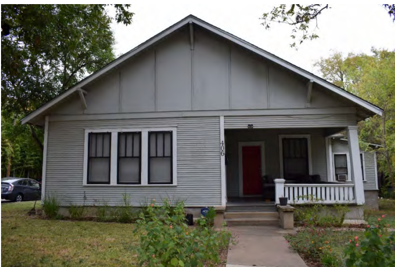
Figure 5-11-5. Façade of the bungalow at 406 West 30th Street (1925). Source: HHM, 2019.
