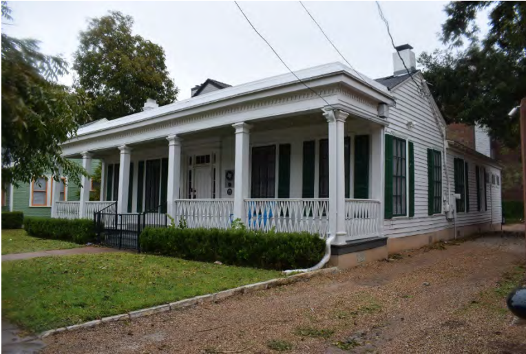
Fig. 4-2-6. Photograph of a 1900 Classical Revival house at 2605 Salado Street. Note the dentils and column capitals, inspired by Greek classical architecture. Source: Photo by HHM, 2019.
