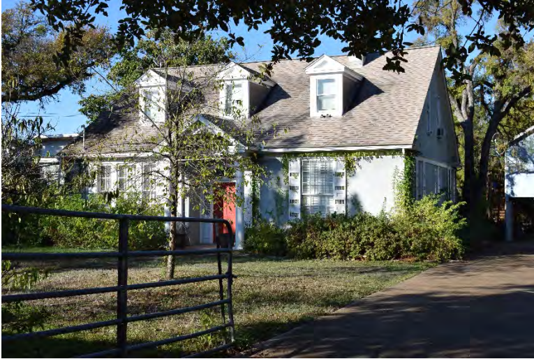
Fig. 4-1-11. This residence, located at 2816 San Pedro Street, is an example of a Cape Cod house . Constructed in 1927, the house has a rectangular footprint, a steep side-gabled roof, gabled dormers, and Classical Revival stylistic influences, all common character-defining features of the Cape Cod form. Source: Photo by HHM, 2019.
