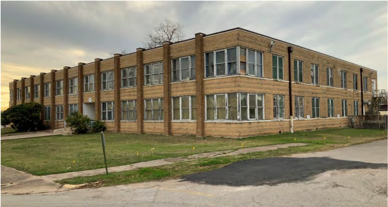
Figure 5-3-8. Oblique view of the ca. 1936 African American Women's Ward (Building 519), demolished in 2020. This is one of the few buildings constructed on the hospital campus specifically to serve the segregated patient population. Source: HHM, 2019.
