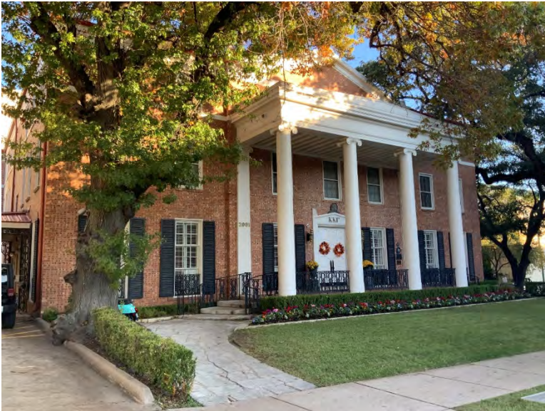
Fig. 4-2-1. Photo of house at 2001 University Avenue. The Greek Revival style is visible in the temple-front portico entrance, Classical porch columns, and front-gabled pediment. Source: Photo by HHM, 2019.
