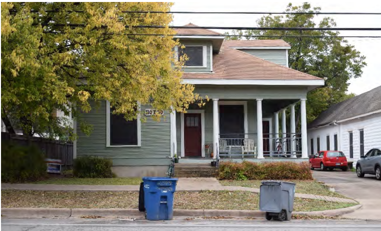
Fig. 4-1-7. This house at 110 E. 30th Street is an example of the modified square-plan hipped-roof plan . Constructed in 1916, this dwelling features similar characteristics as a square plan hipped-roof house—a hipped roof with a centrally located, low-pitched hipped-roof dormer on the front—except it has an inset porch underneath the roofline. Source: Photo by HHM, 2019.
