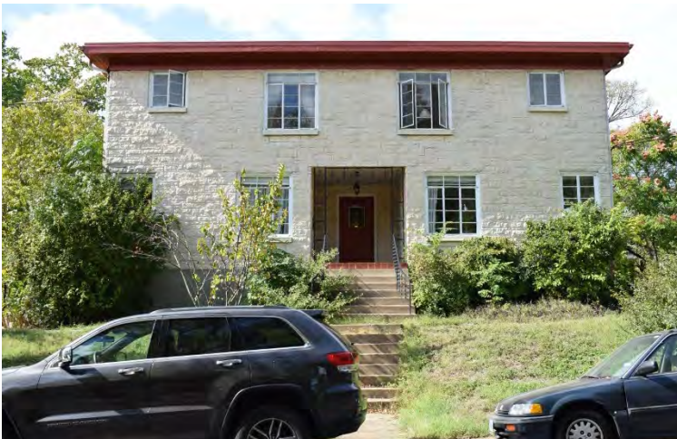
Figure 5-6-11. Façade of the apartment building (1948) at 3300 Tom Green Street. Source: HHM, 2019.
