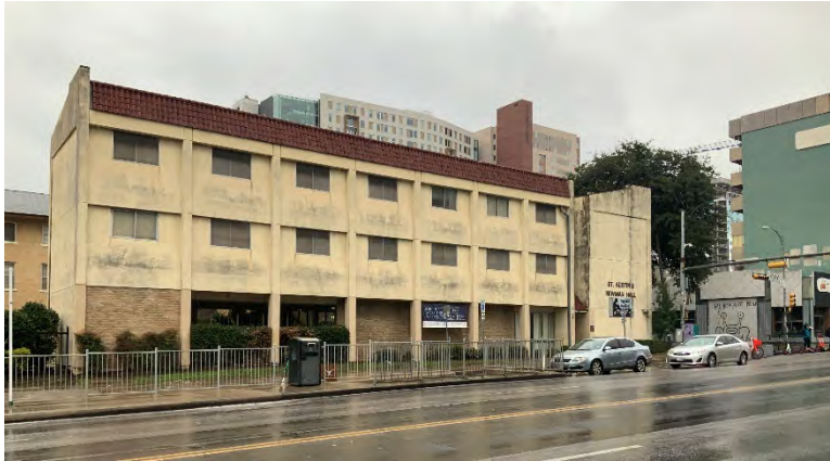
Fig. 4-1-40. This building, located at 2026 Guadalupe Street, is an example of an auxiliary religious building . Constructed as a dormitory for the Catholic Church in 1914 and modified in 1977, the building—known as Newman Hall—is located directly adjacent to the church and has Mission Revival and Mid-century Modern stylistic influences. Source: Photo by HHM, 2019.
