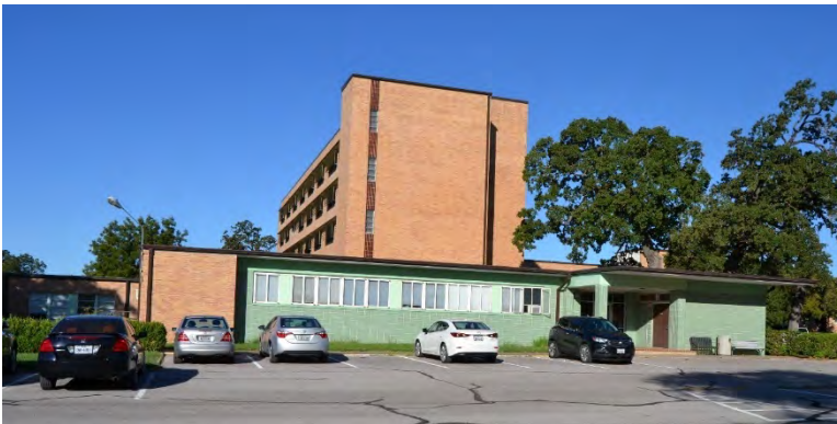
Fig. 4-2-17. Mid-century Modern building on the Austin State Hospital campus. Note the flat roof, unadorned wall surfaces, and horizontal ribbons of windows in the 1955 building. Source: Photo by HHM, 2019.
