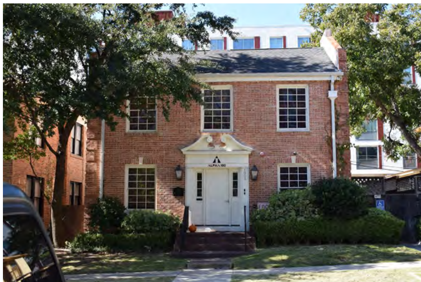
Figure 5-1-23. Small two-story apartment house at 1904 Nueces Street (built around 1930). Source: HHM, 2019.
