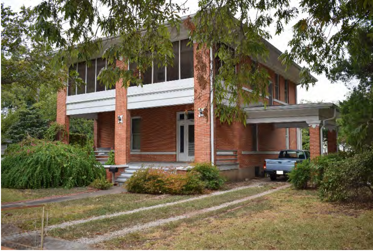
Fig. 4-1-8. Example of a foursquare house located at 4600 Caswell Avenue. This house, constructed in 1920, has many features typical of the foursquare form, including a low-pitched hipped roof, two stories, a prominent, full-width porch, and an offset entry. Source: Photo by HHM, 2019.
