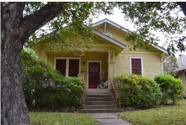
Fig. 4-1-9. This bungalow , at 2825 Salado Street, was constructed in 1923 and showcases several common features of the building type. Key hallmarks of the Craftsman style are also on display, including decorative brackets, exposed rafter tails, and box columns supporting the front porch. Source: Photo by HHM, 2019.
