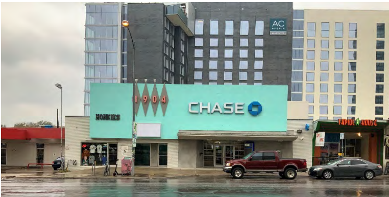
Fig. 4-1-36. This is an example of a bank in the North Central Austin survey area. Constructed at 1904 Guadalupe Street in 1948, it features a one-direction drive-way leading to a canopy where bank transactions with bank tellers took place through windows. Source: Photo by HHM, 2019.
