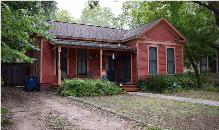
Fig. 4-1-4. This L-plan house is located at 4506 Avenue C and was constructed in 1910. The one-story dwelling displays many typical features of L-plan type houses, including its projecting front-gabled wing and cross-gabled roof. Source: Photo by HHM, 2019.
