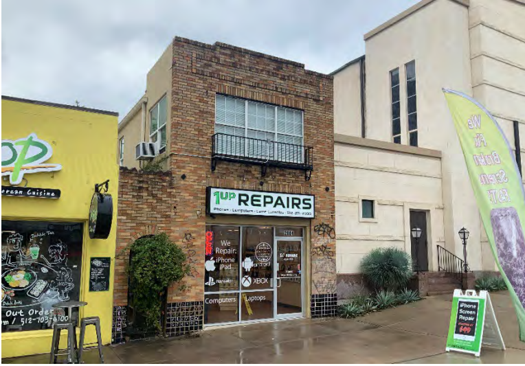
Fig. 4-1-31. Example of a two-part commercial block building at 2004 Guadalupe Street. Note the large storefront windows on the ground floor, contrasted with the second floor's more private windows. Although the original storefront has been replaced, it still echoes the traditional pattern of a two-part commercial block building, with an entrance into the ground-floor retail space at the center of the front façade plus a second entrance leading to the upstairs space at the side (left). Source: Photo by HHM, 2019.
