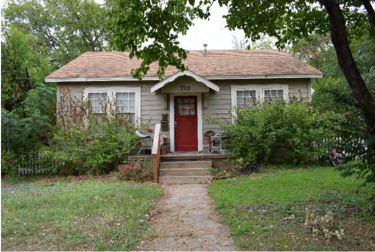
Fig. 4-1-10. This bungalow , at 710 W. 35th Street, was constructed in 1932. The rectangular footprint, side-gabled roof, and portico are typical of the compact version of the bungalow form – which still features parallel interior divisions of bedrooms versus living room-dining-room-kitchen. This example uses the Minimal Traditional style, typical of Austin bungalows from the 1930s onward. Source: Photo by HHM, 2019.
