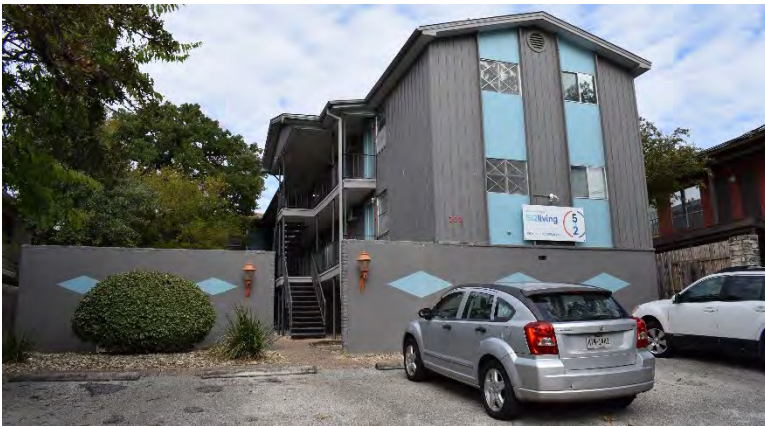
Fig. 4-1-25. This example of a linear mid-rise apartment building is located at 302 E. 34th Street and was constructed in 1972. The long, rectangular building has a linear configuration with balconies facing the front and staircases at each end. Source: Photo by HHM, 2019.
