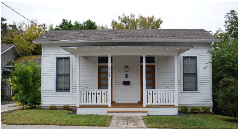
Fig. 4-1-1. This hall-and-parlor house at 621 W. 30th Street was constructed in 1922 and reflects many key traits of the form, including offset entryways, a side-gabled roof, and single-story massing. Though its doors have been modernized, its form remains historically accurate. Source: Photo by HHM, 2019.
