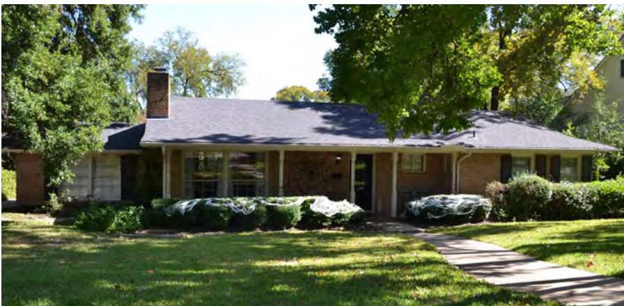
Figure 5-1-29. Example of infill Ranch-style residential construction at 2903 Oakhurst Avenue (1953). Source: HHM, 2019.
