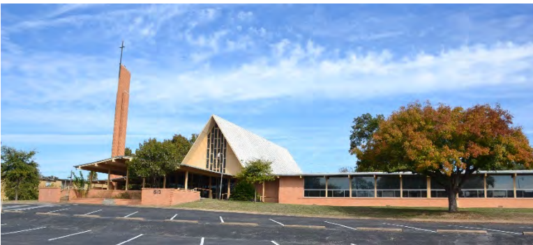
Fig. 4-1-39. Hyde Park Christian Church at 610 E. 45th Street is an example of a Mid-century Modern church in the North Central Austin survey area. This church was constructed in 1959. Source: Photo by HHM, 2019.
