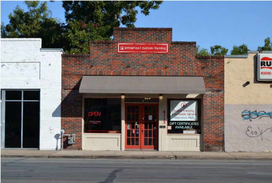
Figure 5-5-4. Façade of one-part commercial block building 4113 Guadalupe Street (1920). Source: HHM, 2020.
