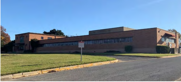
Fig. 4-2-16. A building constructed in 1950 on the Austin State Hospital campus. This building's primary stylistic influence is International style, evident in the flat roof, flat wall planes, and extensive ribbon windows. Source: Photo by HHM, 2019.
