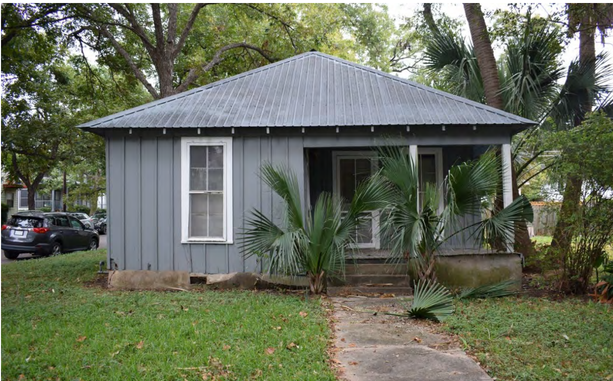
Figure 5-5-2. Façade of square-plan hipped-roof house at 4315 Avenue A (1921). Source: HHM, 2019.
