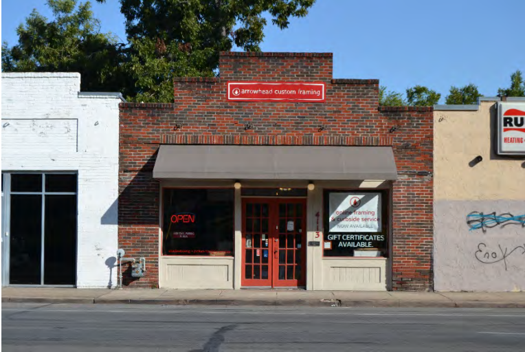
Fig. 4-1-29. Example of a one-part commercial block at 4113 Guadalupe Street. Note the positioning of the building flush with the lot line, the three-part configuration of the front façade, the large windows with transoms, and the prominent sign. Source: Photo by HHM, 2019.
