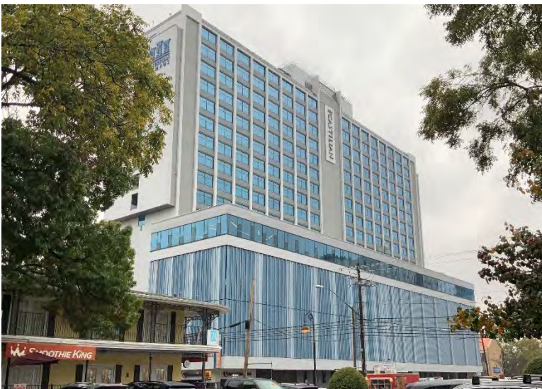
Fig. 4-1-26. Example of a high-rise apartment building at 2323 San Antonio Street, the Castilian Apartment Building, constructed in 1967. Source: Photo by HHM, 2019.
