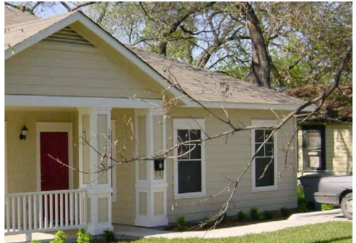
This lot was graded so a flat sidewalk could connect driveway and front door with a no-step entrance instead of a ramp.
