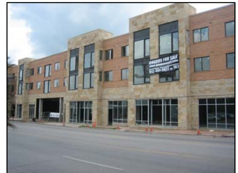
Figure 5-3: Shows façade articulation with a change in plane and also change in color and material.
