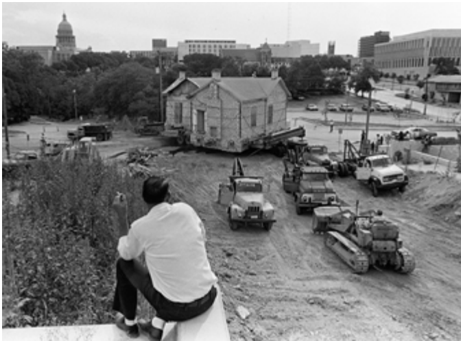
Relocating the 1850s-era William P. Hardeman House from its original location at 401 E. 16th Street to Symphony Square in 1977.
